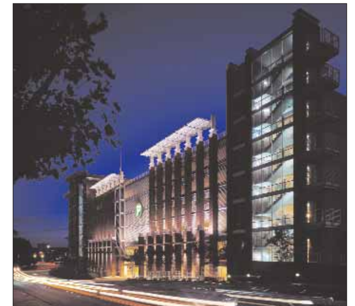
Spring Street Garage & Residential Development – Greenville, SC
